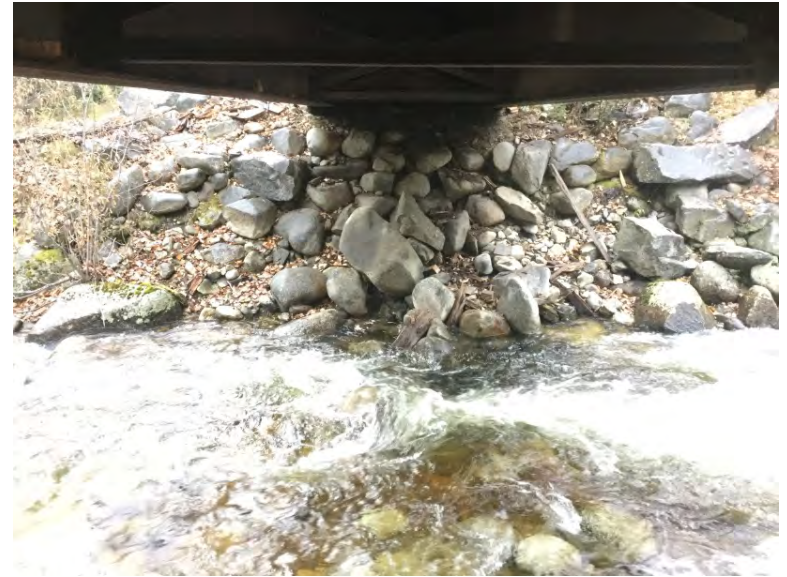
Right Bank Abutment when facing downstream
