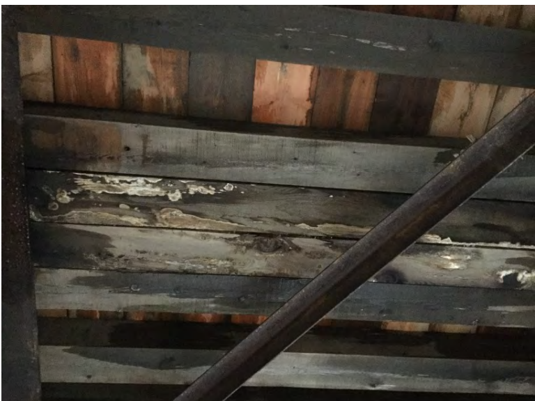
Only subdeck and planks were recently replaced
