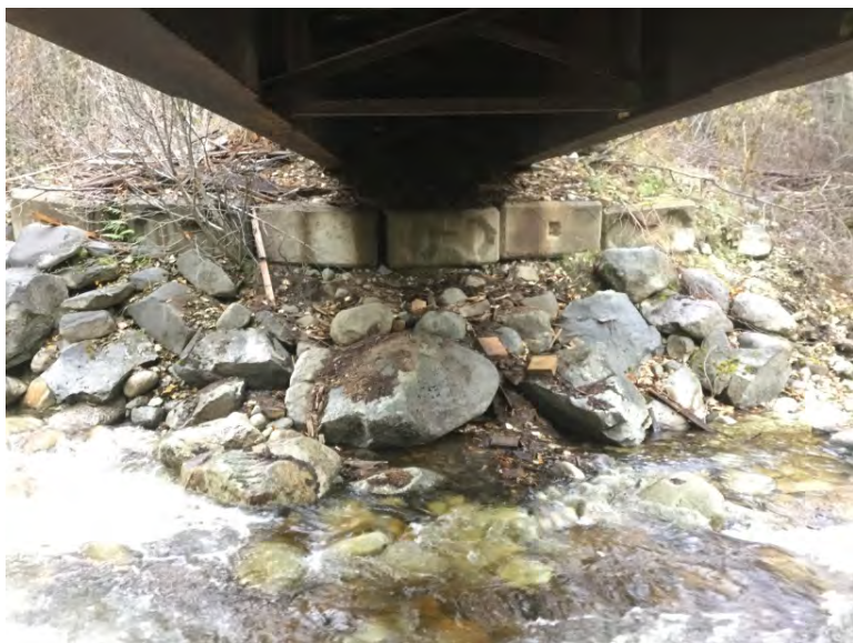
Left Bank Abutment when facing downstream
